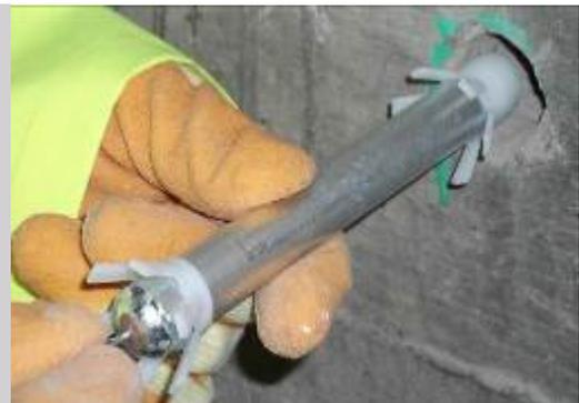
Once the initial charge period was complete each zone was connected in galvanic mode by connecting the anode array directly to steel via the field wiring provided in the local junction box enclosure.
